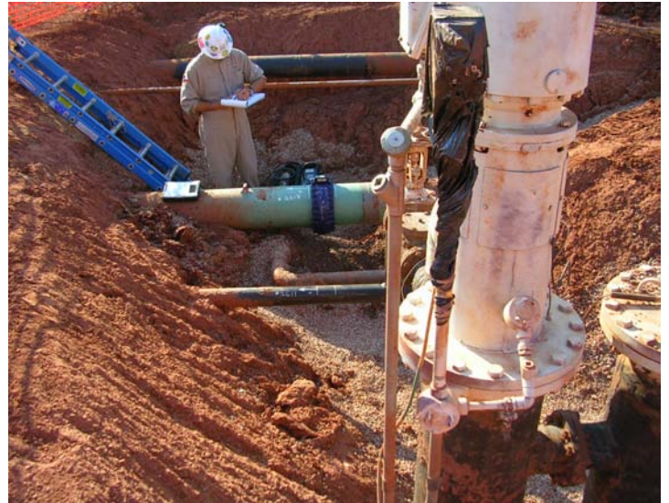
Complete inspection of 112' up-stream and 97' down stream in refinery excavation
