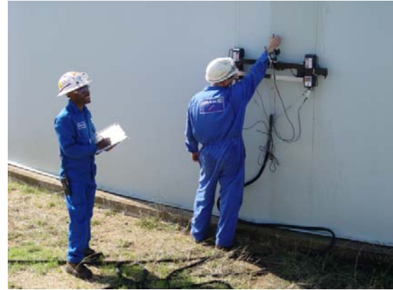
Inspection using LSI™ System is performed by qualified inspector
