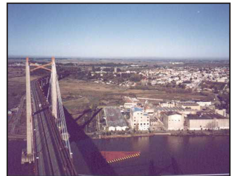
Figure D1: Cable-stayed bridge in Brazil.
