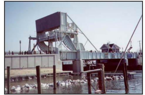
Figure F1: Bascule bridge that was monitored with AE during operation
