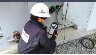
Transformer Clinic's™ **SCREEN** spot inspection services provide an advanced level of instantaneous fault detection and location capabilities. A unique and purposeful range of advanced field-inspection techniques are utilized in a series of real-time spot checks to identify hot-spots and areas of concern.
