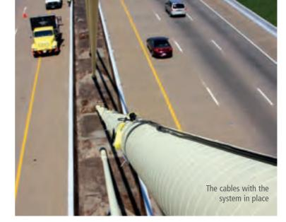
temperature extremes. In addition, this study will evaluate signature sounds and/or wire breaks that occurred during test periods. If cables are found to be acoustically inactive, the system can be moved to another bridge at the end of the monitoring period.
