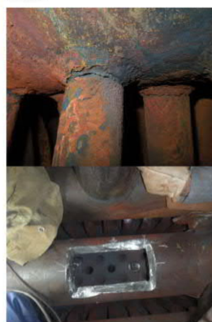
Tube No: 7 on Header 27 with a Crack & Tube Plug with Header Window Cutting Method
