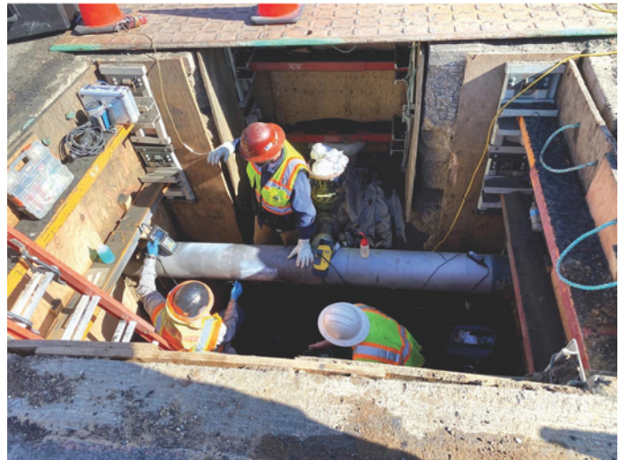
Figure 1. In-situ non-destructive testing is the preferred method for gathering the data required to reconfirm maximum allowable operating pressure (MAOP).
