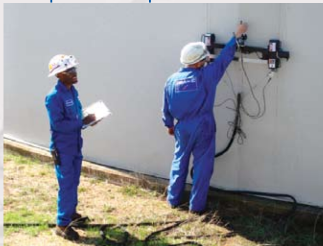
Automated ultrasonic thickness inspection utilizing the LSI System.
