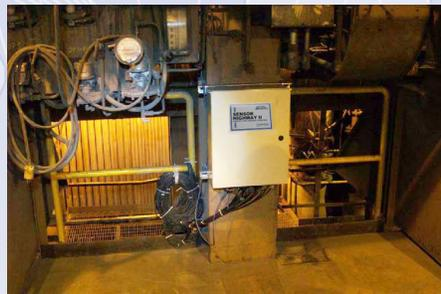
CFM monitors changes in flow and particle size as it impacts the feeder tube and unique, proprietary analysis evaluates the Coal Flow Factor as it changes over time. Unlike other technologies, Coal Flow Factor can detect, identify and differentiate between roping and other adverse changes.
