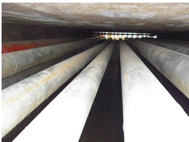
Figure 9a. Pipelines in a road crossing with no access, which were otherwise not tested but with GW they were 100% scanned.
