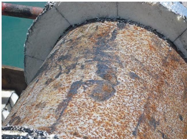
Figure 8. Only 0.5 m of insulation must be stripped to the test position.
